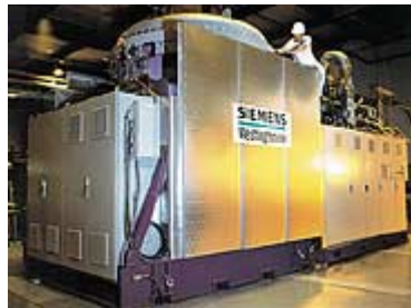
Fig. 47 A 220-kW hybrid system with a Solid Oxide Fuel Cell (SOFC) generator integrated with a micro gas turbine demonstrated at the University of California, Irvine and sponsored by Southern California Edison [Siemens web site]
