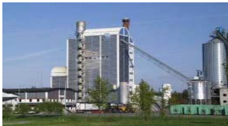
Fig. 26 The Vaxjo Varnamo facility generating 6MW electricity and 9MW of heat from dry biomass
