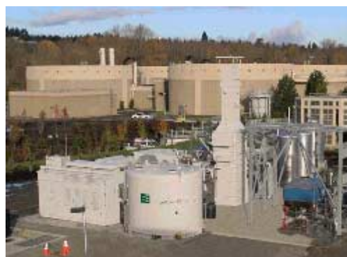
Fig. 13 A 1-MW MCFC of FuelCell Energy [Fuelcell Energy Inc. web site]
