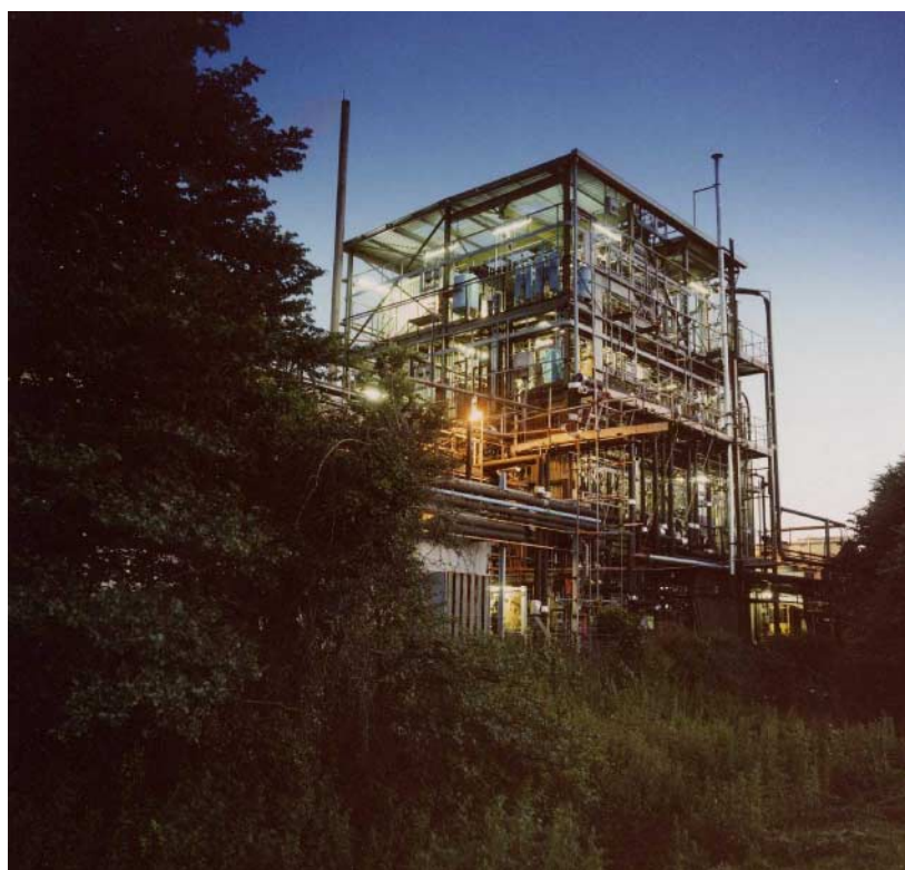
Figure 9. The British Coal Corporation 5 MW th fluidised bed gasifier, used to successfully co-gasify coal and sewage sludge.
