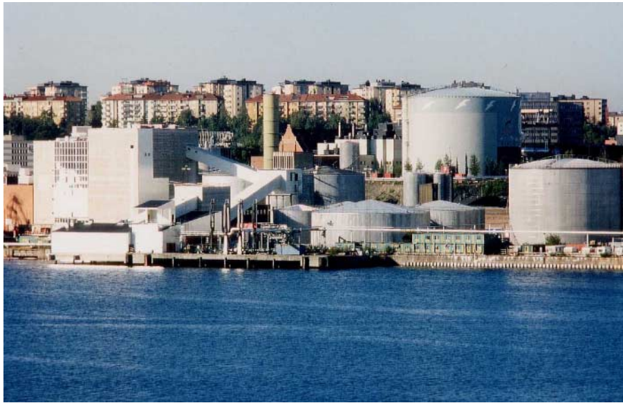
Figure 8. The Vaertan PFBC-based CHP plant, Stockholm.
