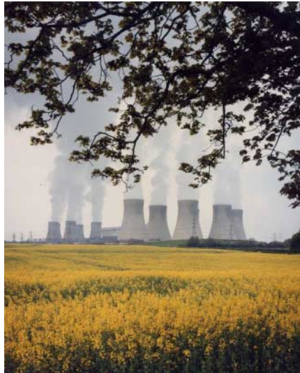
Figure 2. Drax Power Station, United Kingdom
