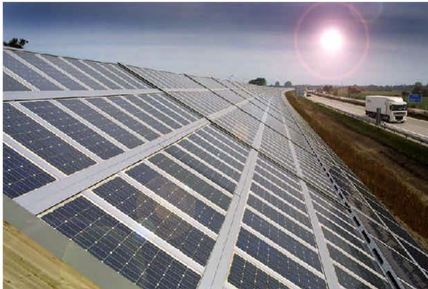
PVSoundless PV Sound barrier at Freising
