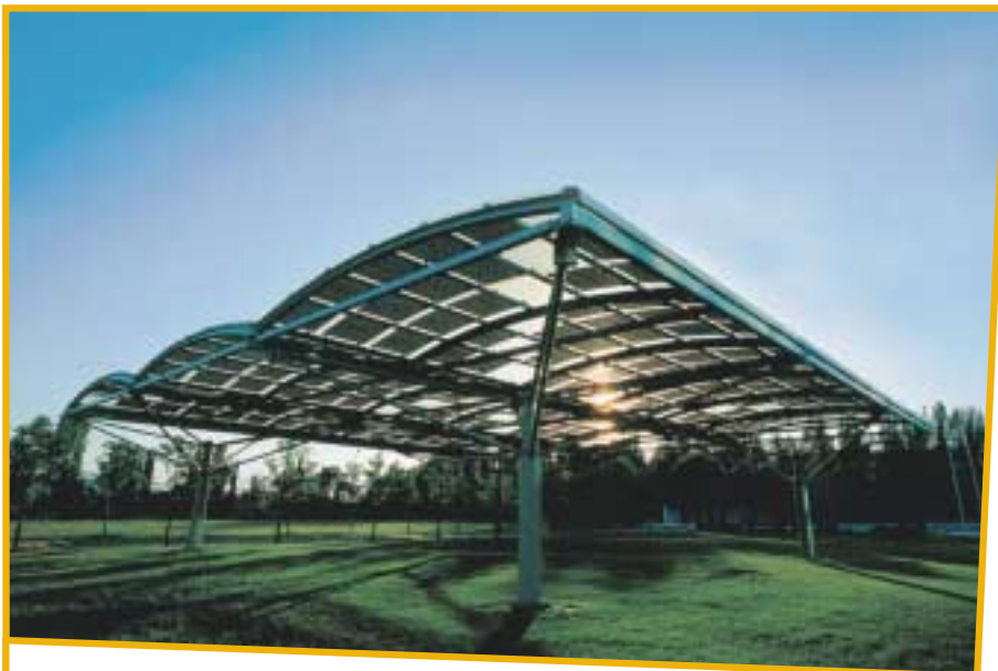
Solar photovoltaic pergola at “La Moncloa” (the Prime Minister’s residence)
