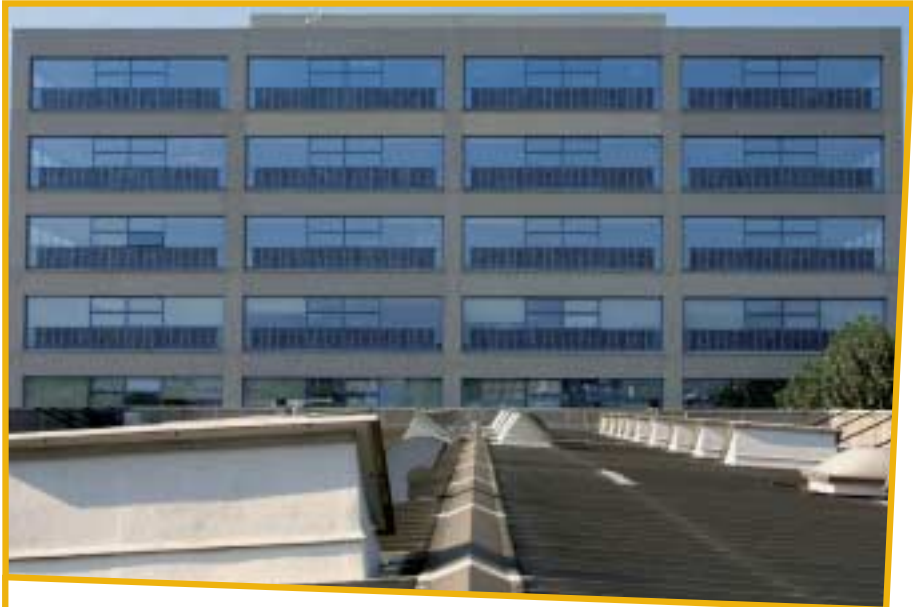
Grenoble building South-East façade
