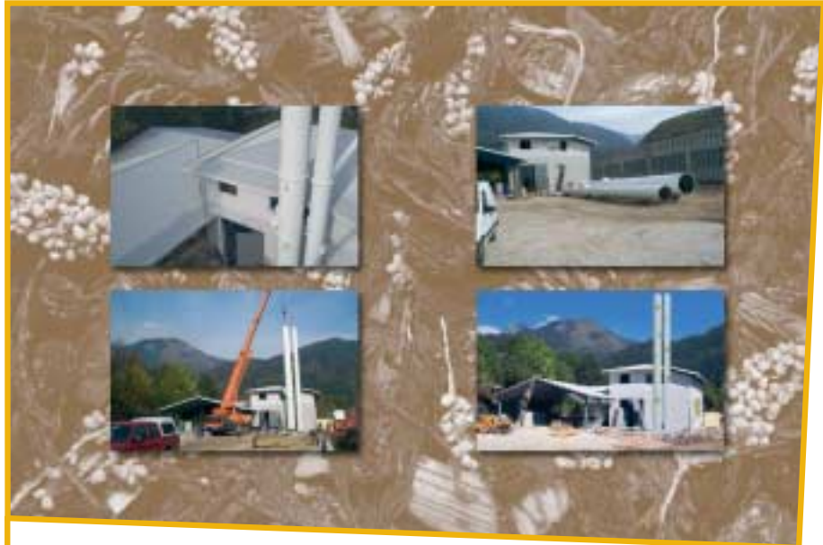
Construction of the district heating system in Predvor
