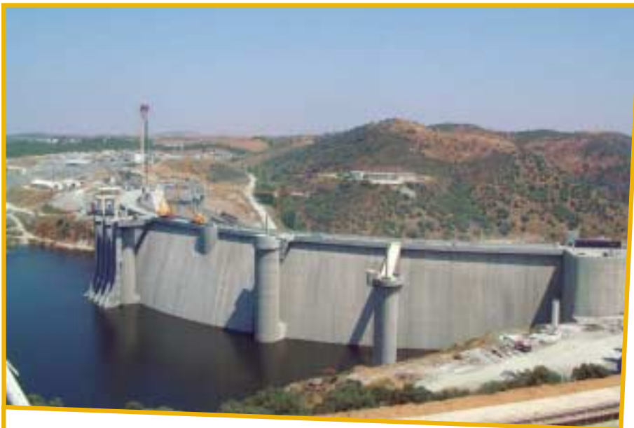
Overview of the Alqueva Dam
