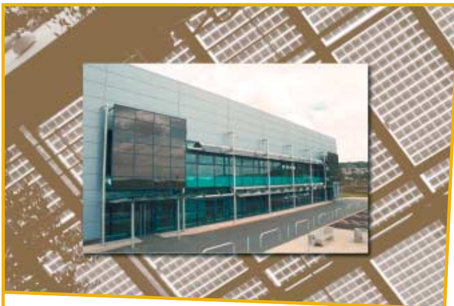
Detail of solar photovoltaic panels
