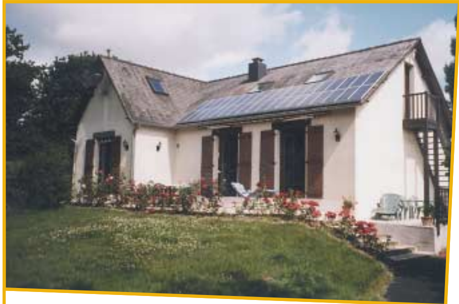
Solar system used in a rural dwelling
