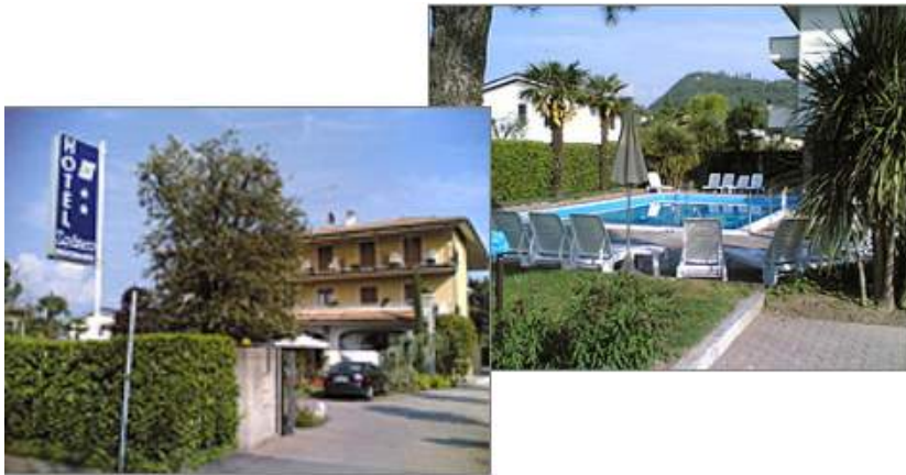
Hotel Zodiaco – Manerba del Garda, Italy, 106 kW heat/51 kW cool
