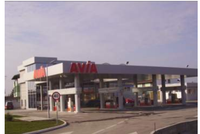
Gas filling station AVIA – Novi Sad, Serbia 135 kW heat, 34 kW cool
