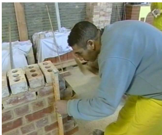
Laying foundation stones for future work
