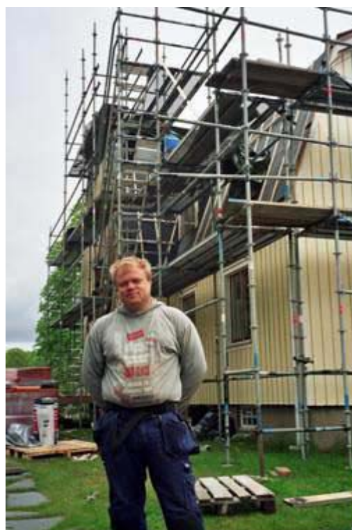
Cook, welder, roofer... Rickard Sörelid reroofs a house at Alingsås
