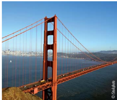
Golden Gate Bridge in San Francisco
