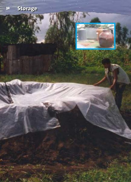
Plastic lined tanks can be a low cost alternative to metal or ferro-cement tanks.
