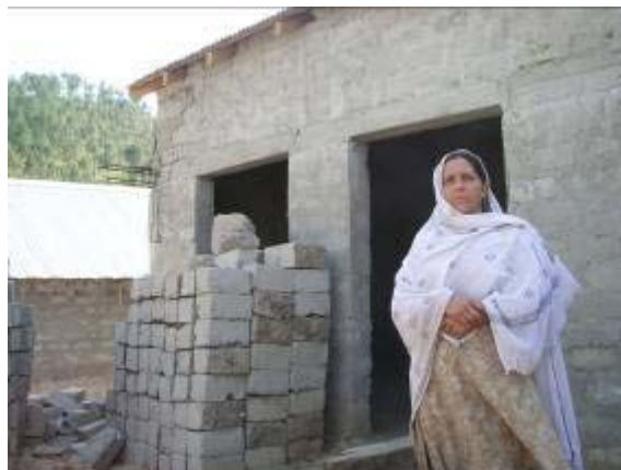
Figure 7: This widow near Mansehra was forced to knock down her half-built house because it did not comply with the latest ERRA guidelines, although it was in compliance with the initial guidelines. (Photo S Nam).
