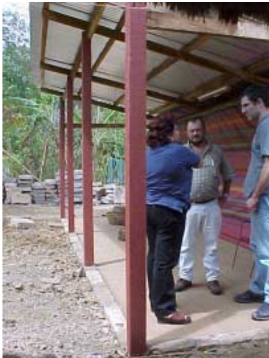
Photo 4 Example of piso-techo construction by ACSUR Las Segovias in Masaya, Nicaragua
