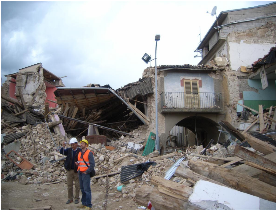
Figure 7: Collapse of old masonry buildings in Onna
