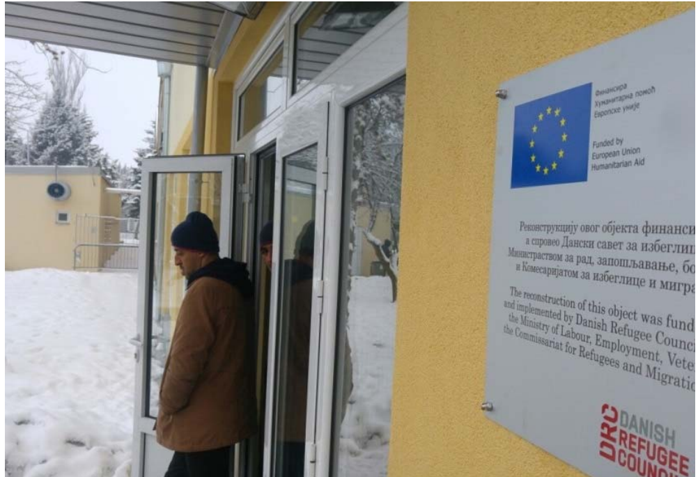
A reception centre for refugees and migrants in Preševo, southern Serbia, which was extensively renovated with EU funds © UNHCR
