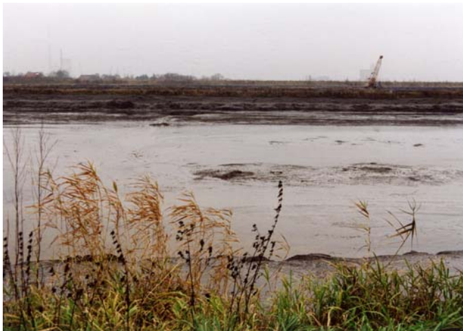
Figure 8: Site visit to the harbour sediment treatment facility in Bremen/Seehausen operated by BremenPorts GmbH & Co. KG- one of several dewatering lagoons for harbour sediment
