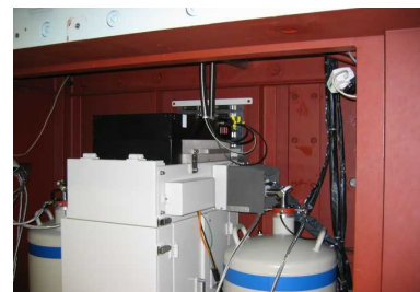
View of a combined X-ray densitometer / neutron counter installation in the On-Site Laboratory at Rokkasho.
