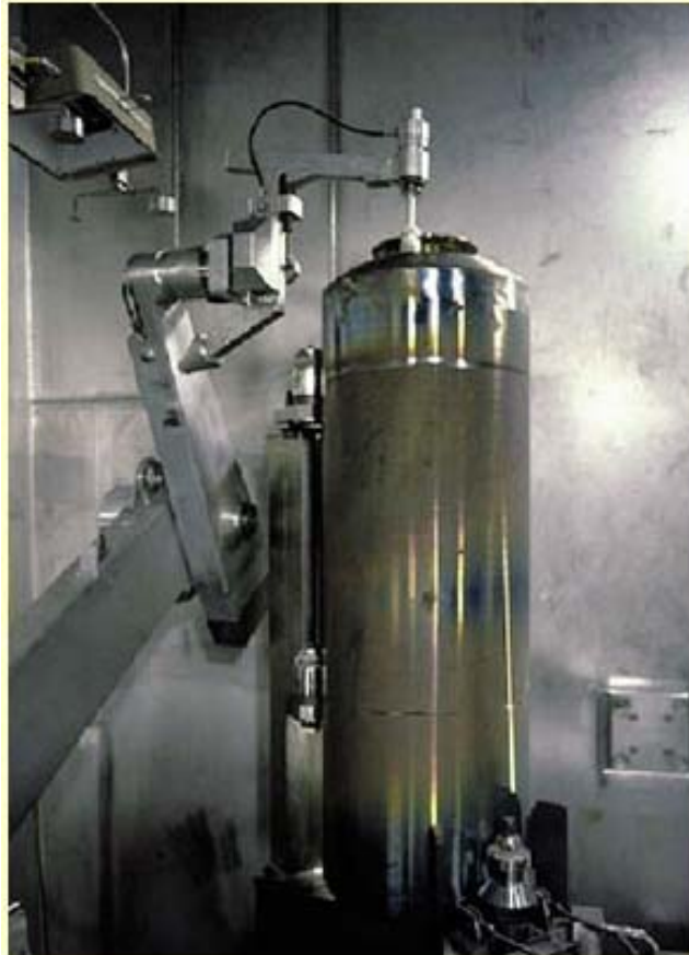
Vitrified waste canister being inspected in the R7 vitrification facility in the Cogema UP2-800 waste-reprocessing plant at La Hague (Manche département). Sidney Jezeque/Cogema
