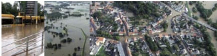
Images taken during the Elbe flood in August, 2002. Aerial photos © pik-postdam.de
