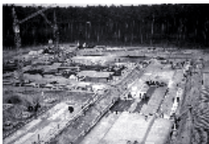
Construction of the ITU in 1963.
