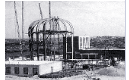
Construction of the HFR reactor, Petten.
