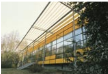
The retrofitted Mensa building (Ispra), February 1996.
