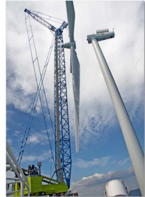
Construction of Lillgrund offshore wind farm, Sweden 2007
